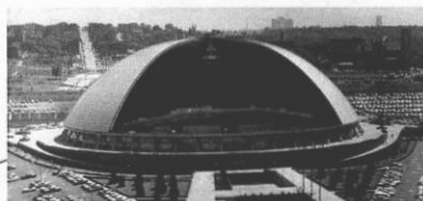
Ammann & Whitney, deployable dome-like roof of the 'Civic Auditorium' in Pittsburgh/PA built 1958-61, demolished 2012
